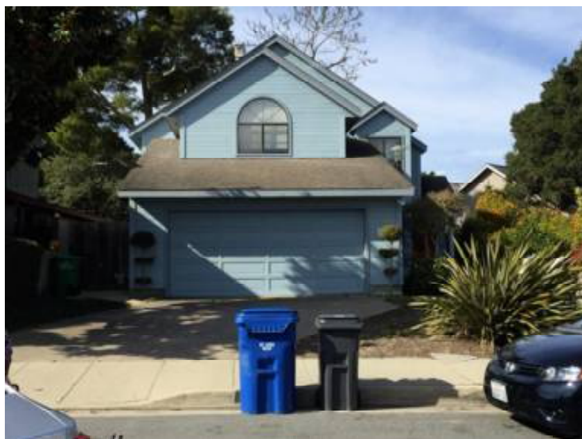
Fig 12. 20 foot setback and two car garage for two story neighboring home at 110 20 th Street
